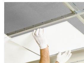
The individual tiles are easily demountable
