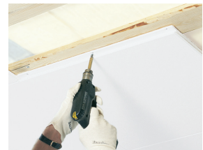
Focus F is installed by screw fixing
