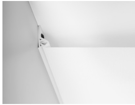
Clipso ceiling installation with PCW profile.
