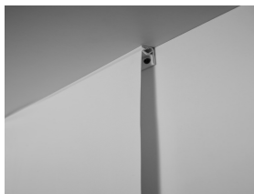
Clipso wall installation with PCC profile.
