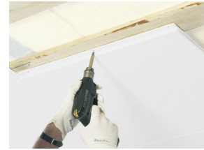
Focus F is installed by screw fixing
