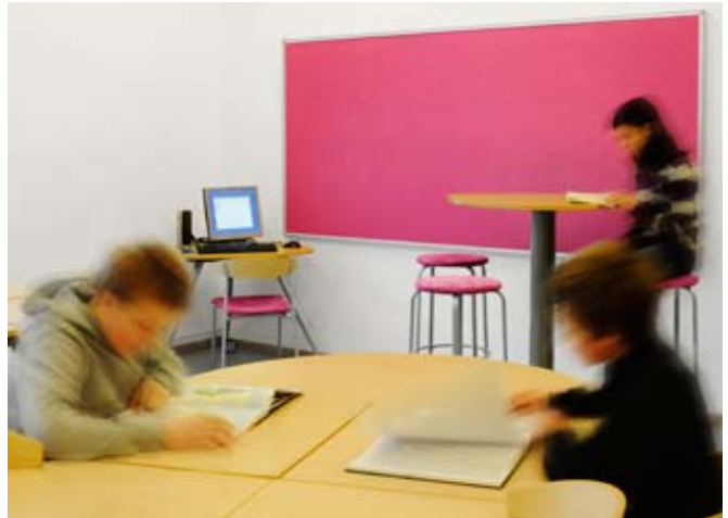
In a classroom, the wall absorber helps to reduce the sound level and remove unwanted sound reflexes.
