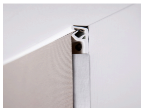
Clipso wall installation with PCC profile.
