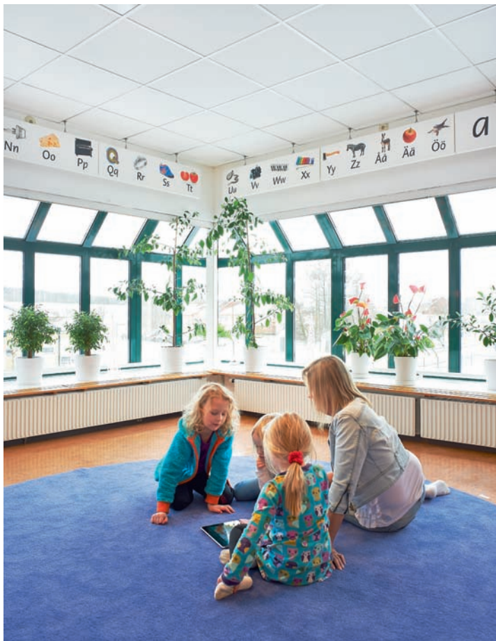
An overall acoustic ceiling combined with printed “pedagogic” sound absorbers in the ceiling angle did the trick.
