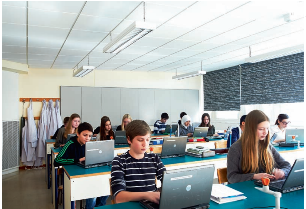
Ecophon Master™ Extra Bass has been installed above the acoustic ceiling, in order to reduce low-frequency sound reflections. Ecophon Akusto™ Wall C in the background. The sound behaves similar to the forest with no disturbing sound reflections which positively affects the speech intelligibility.
