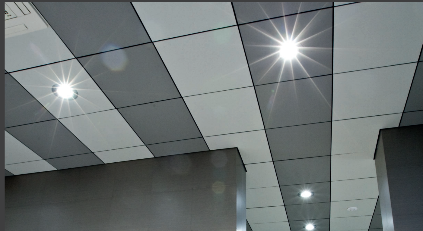
FOCUS Dg Unique edge design with concealed support edges and a floating appearance.
