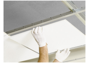
The individual tiles are easily demountable
