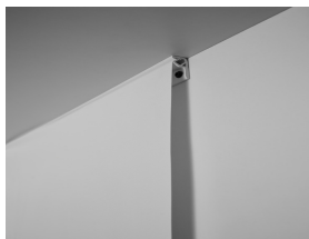
Clipso wall installation with PCC profile.
