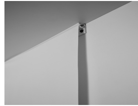
Clipso wall installation with PCC profile.
