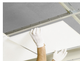
The individual tiles are easily demountable
