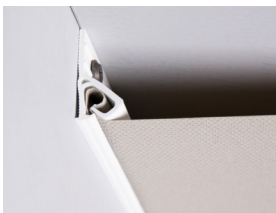
Clipso ceiling installation with PCW profile.
