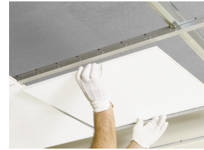
The individual tiles are easily dismountable
