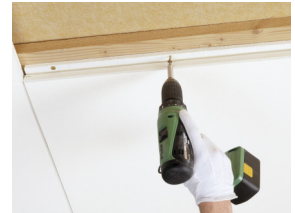
Master F is installed by screw fixing
