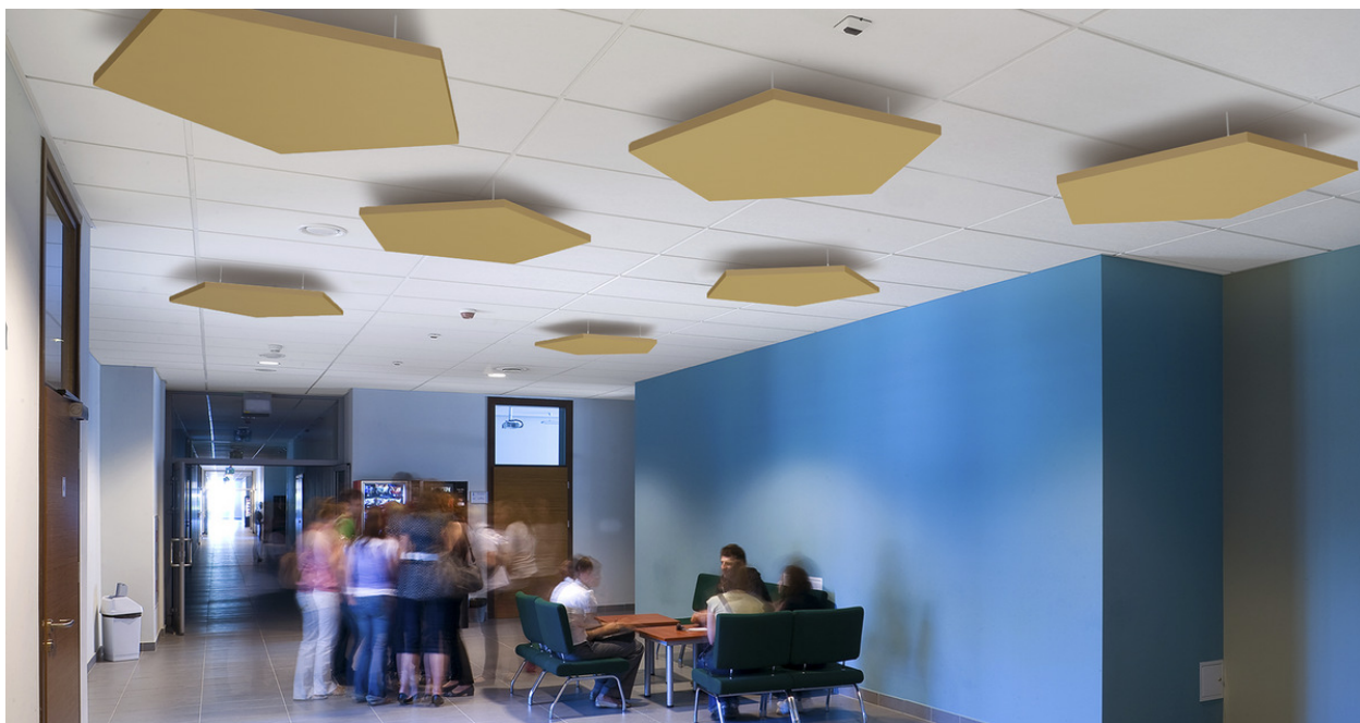
Ghalamco Arena, Belgium
