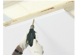
Focus F is installed by screw fixing
