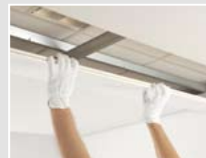
The individual tiles are easily demountable
