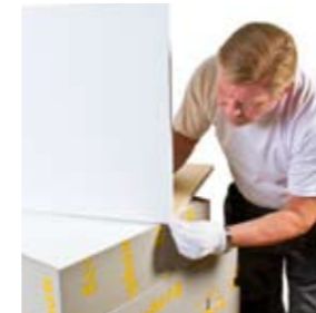
A neat finish To ensure a neat finished result the plug is carefully aligned with the edge of the sound absorber.
