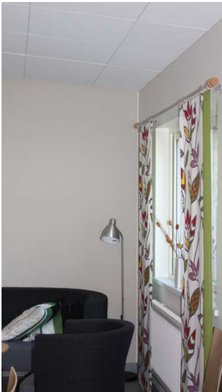
Figure 5. Ceiling absorber: Ecophon Master B
