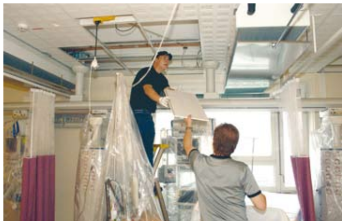
The old suspended ceiling in room 5 was removed and replaced ...
