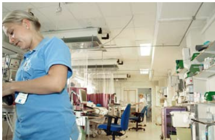
... with a class A acoustic ceiling that reduced the sound level by 3 dB(A) and considerably reduced sound propagation.
