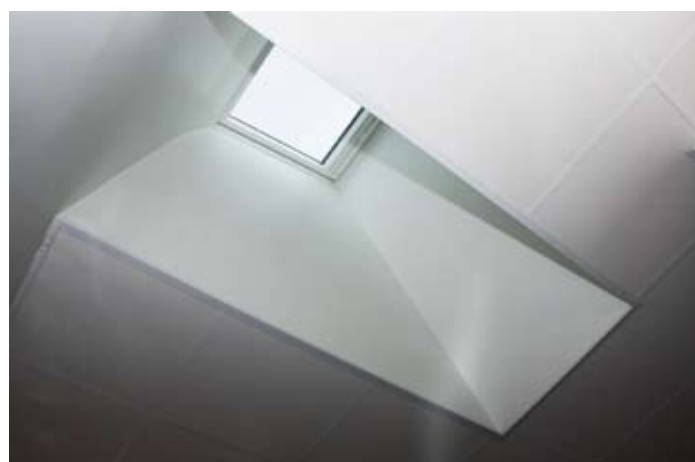
A light well penetrates the full acoustic ceiling. Cleverly placed windows admit as much light as possible without excessive direct sunlight.
