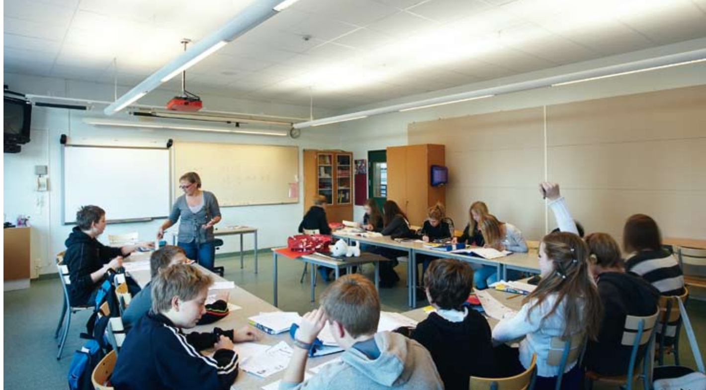
“It’s now much lighter and the acoustic environment is better than before,” comments Frida Wirén, who is seen here teaching year seven pupils. The acoustic ceiling combined with wall absorbers on the right provides the ideal conditions for communication and speech perception.
