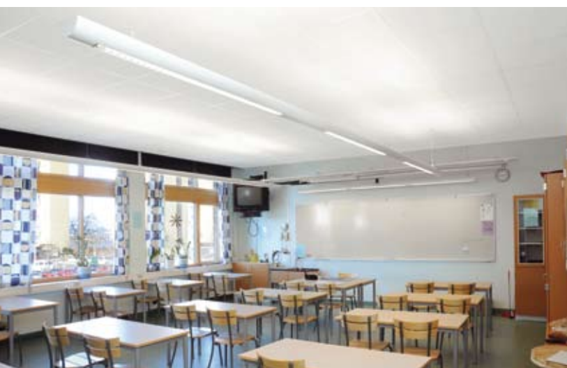
After. Quite a transformation. The uplighters spread uniform light throughout the classroom thanks to the acoustic ceiling’s ability to reflect light without glare. The ceiling meets the highest absorption class, class A, which makes it easier to communicate effectively and allows everyone to hear each other much better.
